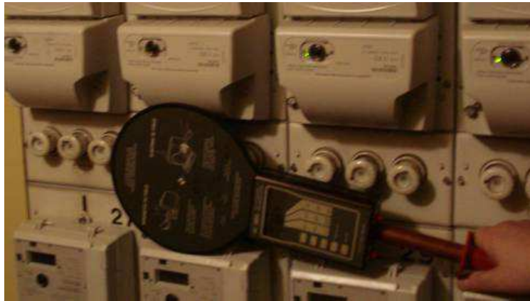
Figure 2: Example of electric field measurements of the basement.
