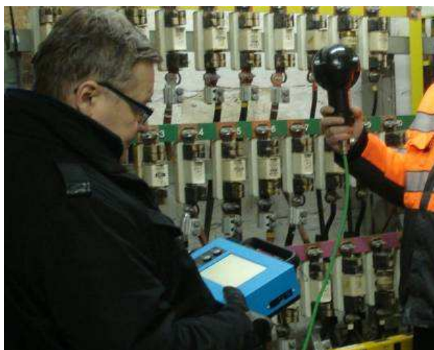
Figure 1: Measurement Place A, near fuse panel.
