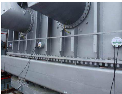
Figure 2: Sensing heads mounted on the transformer.
