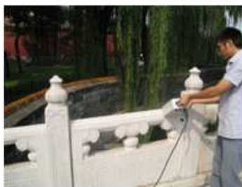
Figure 1: 4 GHz antenna being used on a historic bridge inside the Forbidden City, Beijing.
