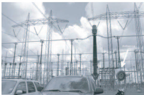
Figure 2: Typical HV equipments in the 735 kV substation.
