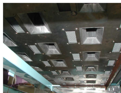
Figure 12: Microwave part of the microwave drying machine.
