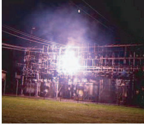
Figure 2: Explosion of a VHV transformer: an example.
