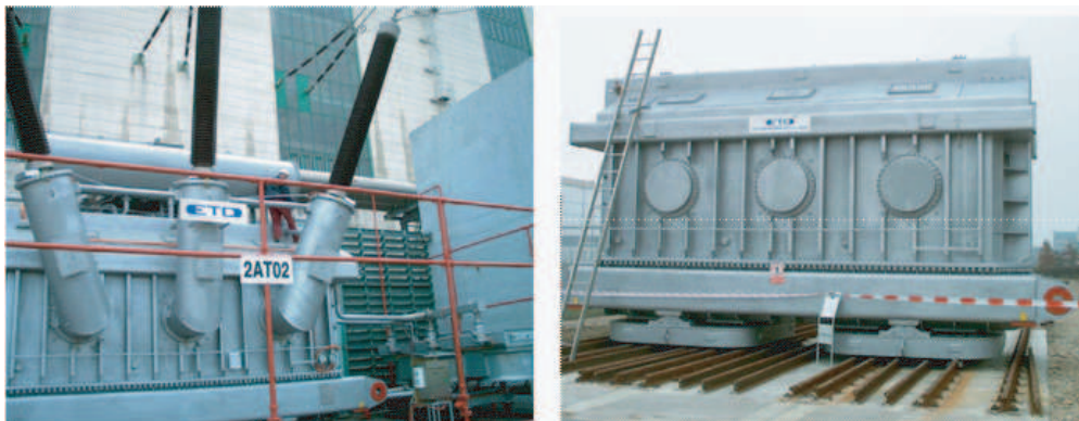
Figure 1: Example of a distribution VHV transformer.
