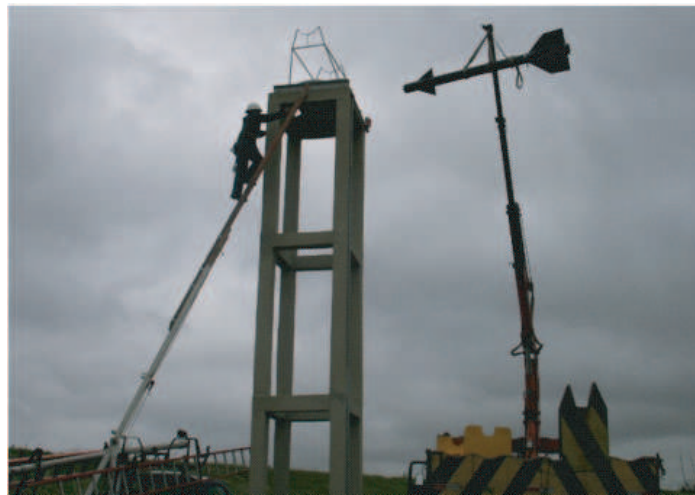
Figure 5: Mounting of a decommissioned air-to-air missile on the pylon with a boom crane.
