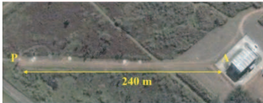
Figure 1: Aerial view of the RCS facility. The positions of the receiving and transmitting radar antennas and the support pylon are indicated by “A” and “P”, respectively. The antennas are located at the corner of the building facing the pylon P. The ground between the antennas and the pylon is composed of compacted soil covered with low vegetation. (Image Google Earth).
