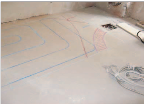
Figure 2: Position of heater tubes was marked by blue chalk, and red chalk was used for cables.
