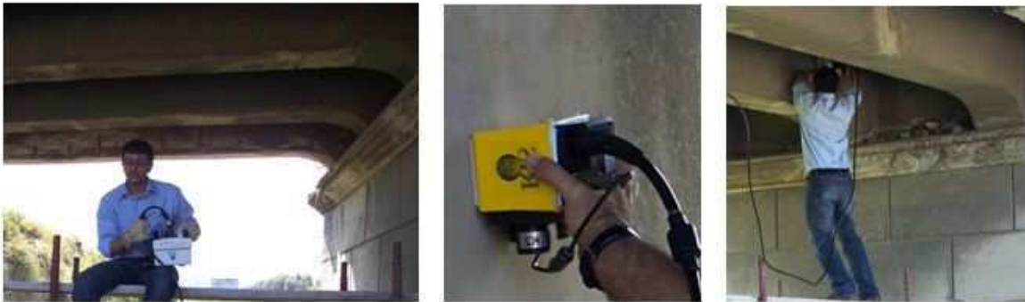
Figure 1: The antennas employed in the survey and an overview of both the bridge and the reinforcement bars “checked” in our testings. In the photograph one of our researchers can be recognized while positioning the measurement instruments on the structure.
